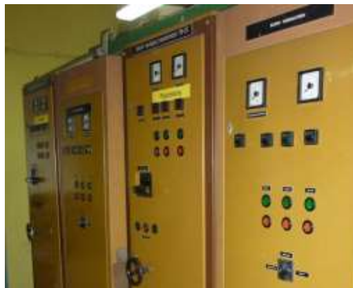
szafy sterownicze (control and measurement equipment)
