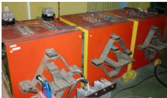
transformatory wielkopiędowe (high current transformers)
