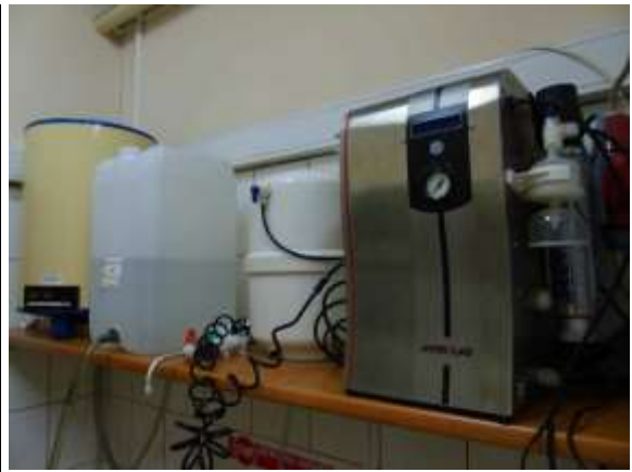
Installation of deionized water
